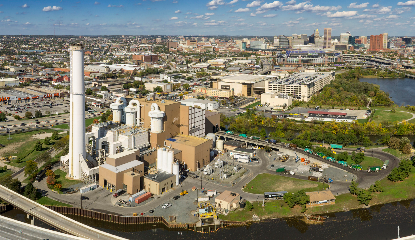
Baltimore waste-to-energy facility
